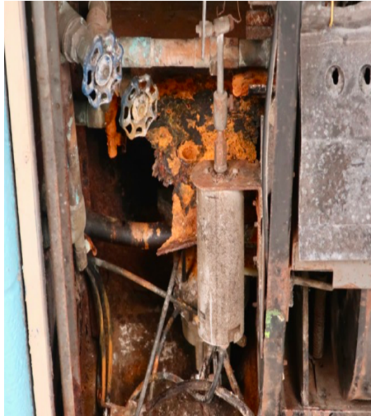
Photo 10 – Elem. Boys Bathroom— Filthy conditions, leaks on floor and ceiling deteriorated/damaged and missing insulation on piping presenting a burn hazard from very hot heating pipes.
